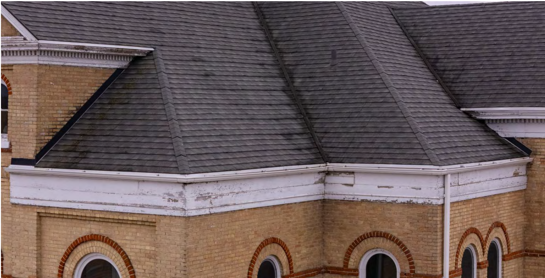
PHOTO - UPPER FRIEZE ROOF
